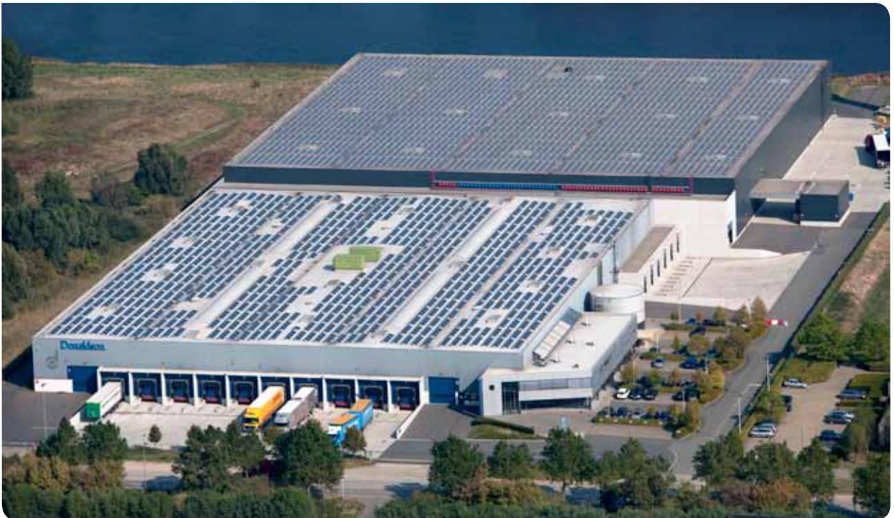
Donaldson Europe - Bruges - Belgium - 970 kWp
